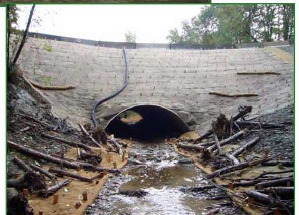
Culvert replaced through the Family Forest Fish Passage Program
